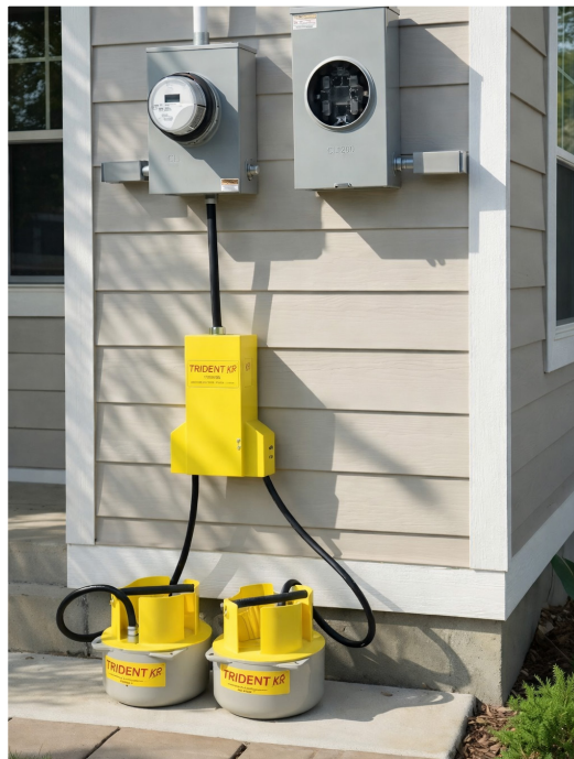
Version B: Direct Wire, Bottom Knockout
