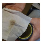
Effectively removes contaminants prior to electrofusion.
